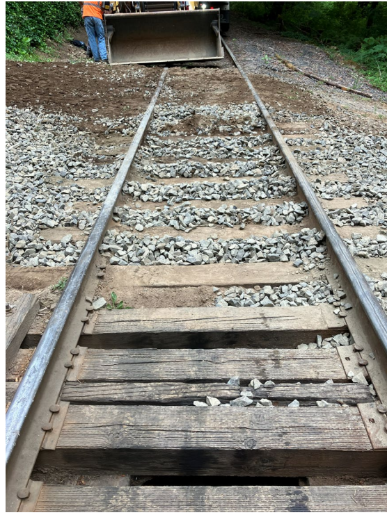
(Correcting a low approach on a bridge.)
