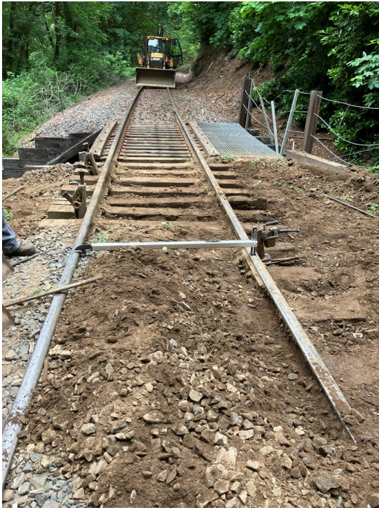
(Correcting a low approach on a bridge.)
