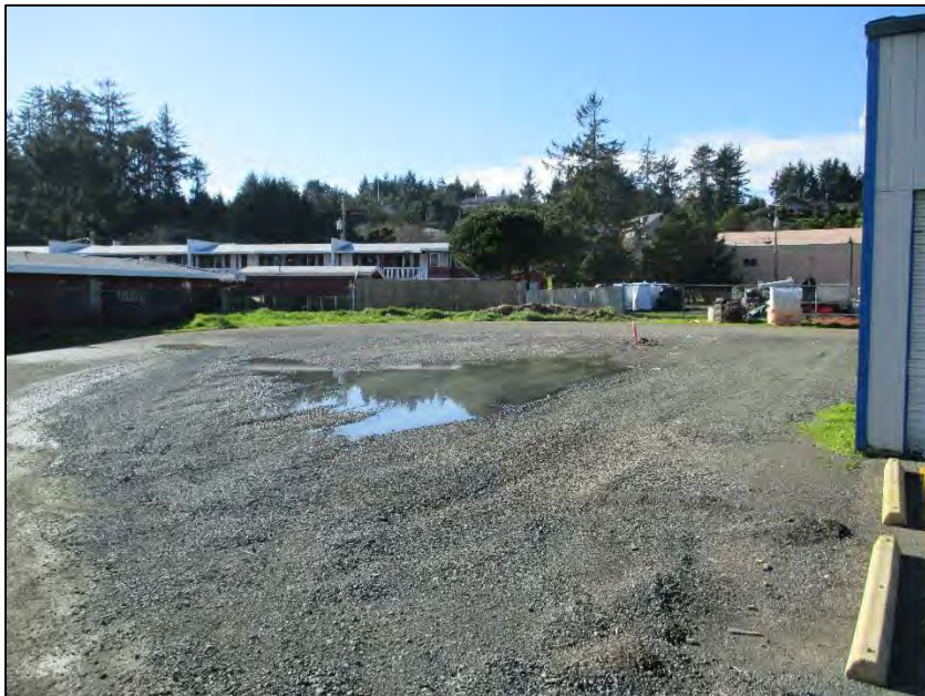
Photo 14. Stormwater ponding at south end
