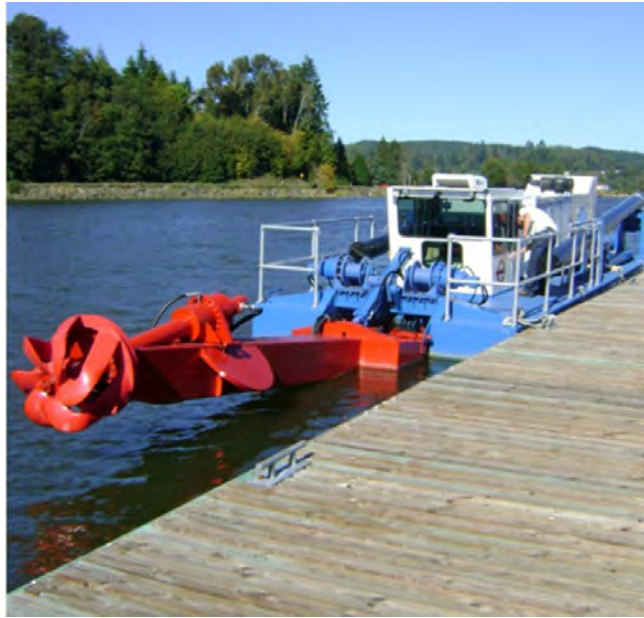
Figure 8. Hydraulic Cutterhead Dredge 370 HP owned by Port of Willapa Harbor, WA
