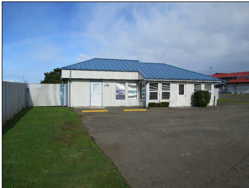
Photo 7. Commercial building on Kingfisher Road
