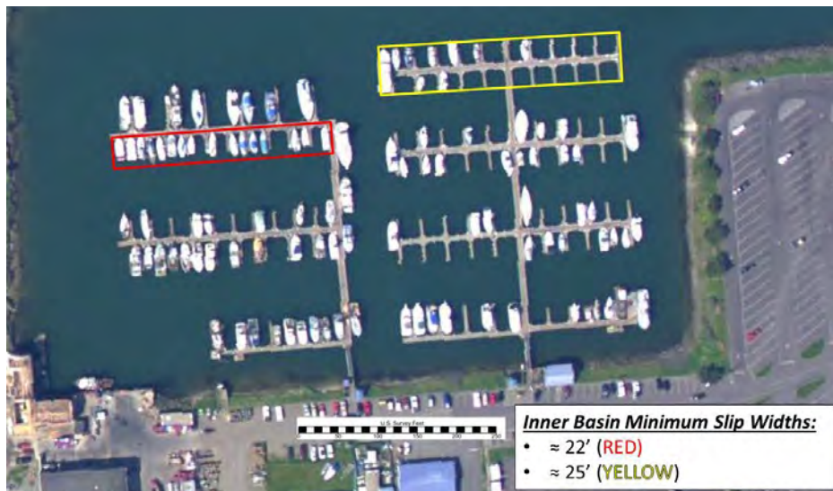
Figure 7. Charleston Marina Inner Basin, measured distance between slips
