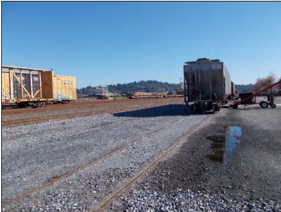
Photo 40. Coos Bay rail yard
