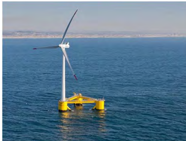
Figure 26 – Floating Wind Turbine
