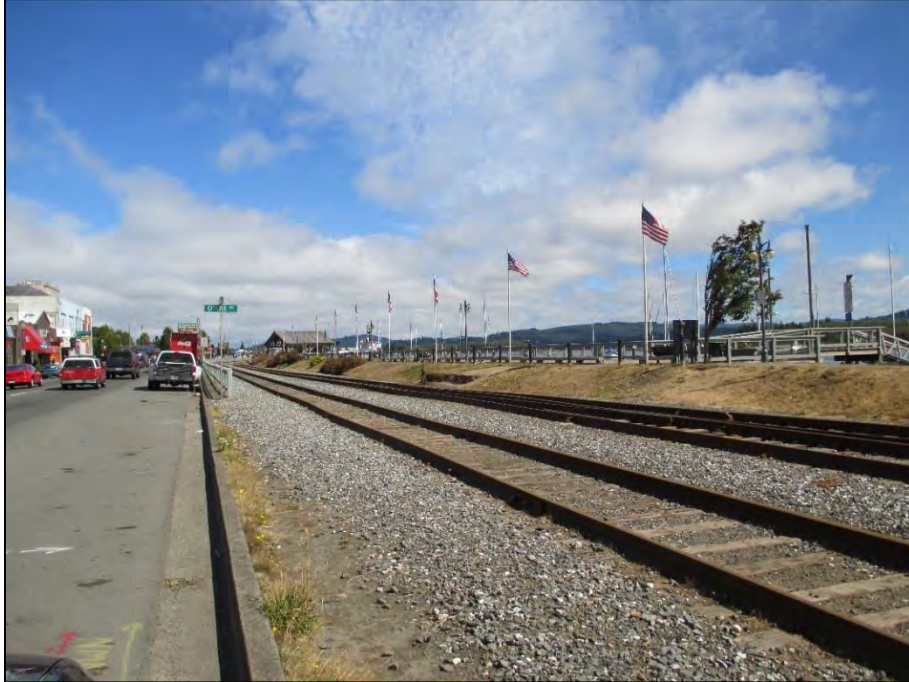
Photo 39. Location of fence extension
