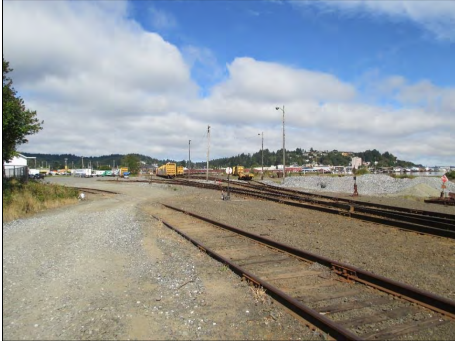
Photo 41. Coos Bay rail yard
