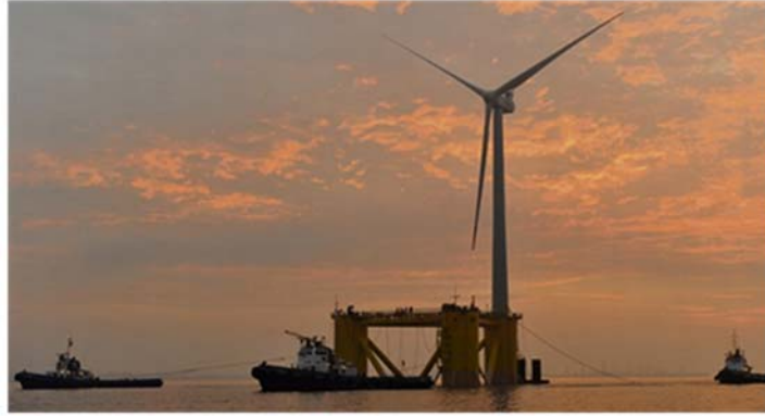
Figure 27 – Floating Wind Turbine
