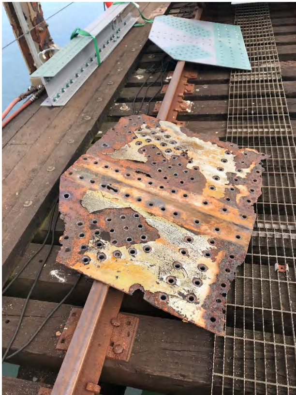
Photos: Work on the North Bend Swing Span repairs. This is the west truss span 6 showing the new base connection plate going in and preparing to install the new vertical member. Photo at left shows the difference in condition of the old versus new plate, and the temporary jacking post in place. Photos taken August 17, 2021.
