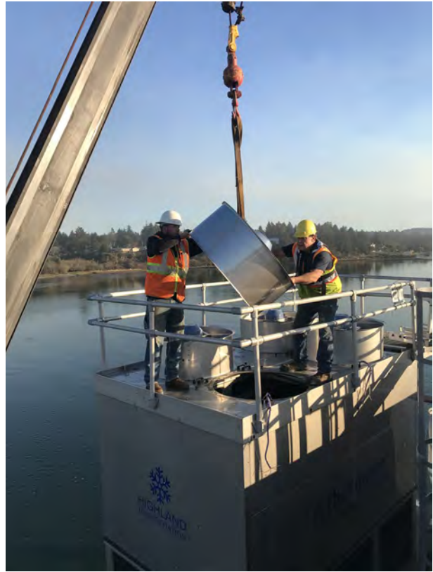
Maintenance Operators Jeremy Beard and Brian Buck assemble and install the new condenser fans for the Charleston Ice Plant using the crane from the Port's boom truck operated by Maintenance Foreman Trent Walker (not pictured).
