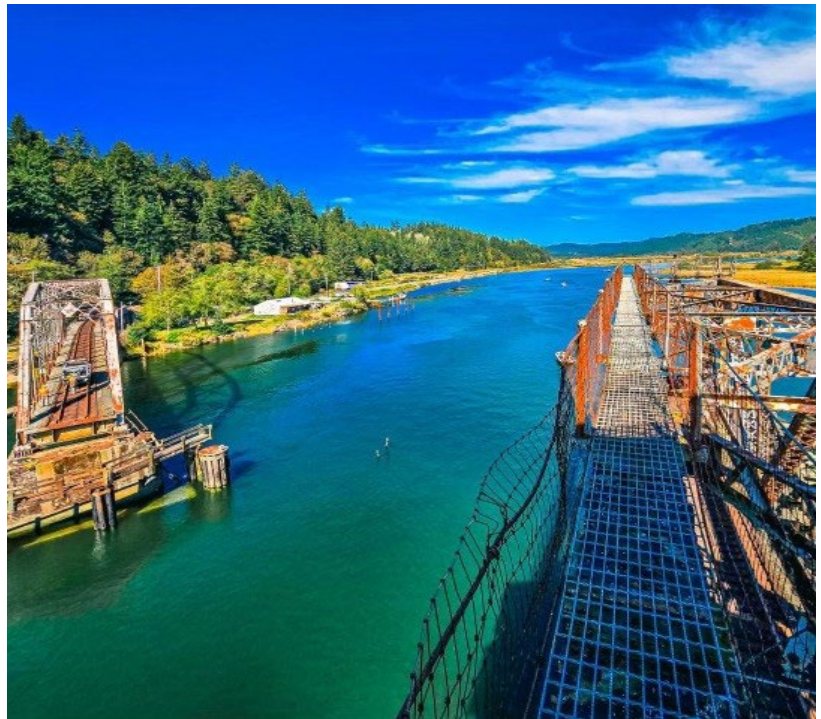
(Cushman swing span in the fully open position, courtesy Rodney Kreidler)
