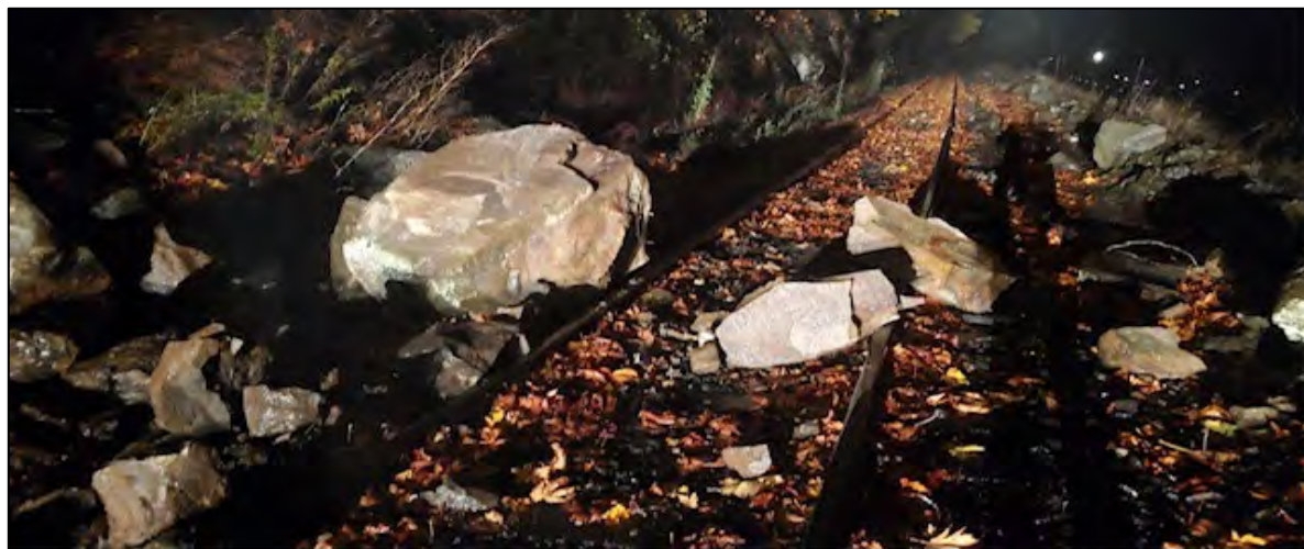
Rockslide at MP 714
