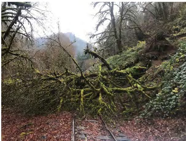
Tree down at MP 685.5 near Richardson Rd.
