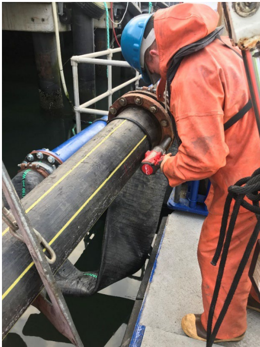
Trent Walker, Maintenance Foreman, and Richard Poetzl, Maintenance Apprentice II, attach pencil buoys to the dredge pipe. These pencil buoys have blinking lights on them so mariners can see the path of the dredge pipe at night.
