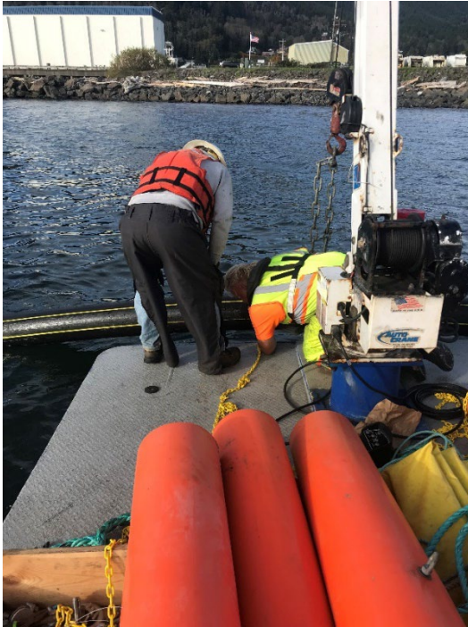
Trent Walker, Maintenance Foreman, and Richard Poetzl, Maintenance Apprentice II, attach pencil buoys to the dredge pipe. These pencil buoys have blinking lights on them so mariners can see the path of the dredge pipe at night.
