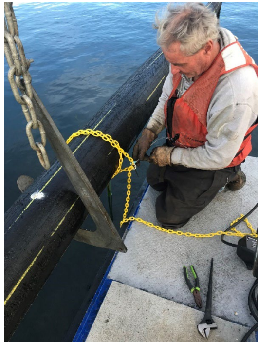
Trent Walker, Maintenance Foreman, and Richard Poetzl, Maintenance Apprentice II, attach pencil buoys to the dredge pipe. These pencil buoys have blinking lights on them so mariners can see the path of the dredge pipe at night.
